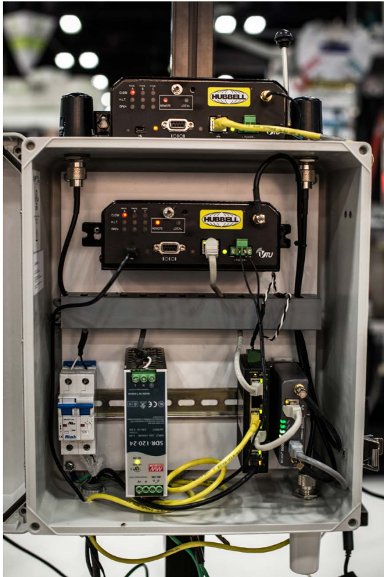
This is a typical field installation, Hubbell only supplies the VTU.
